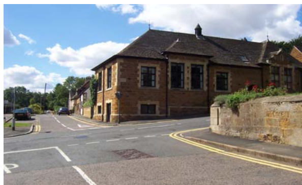
Lack of visibility when emerging from South View
