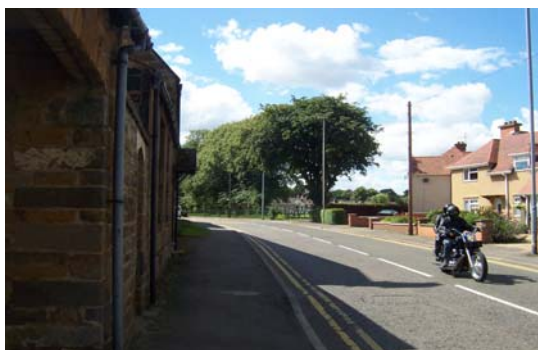
Spot the pedestrian crossing in North Street East ?
